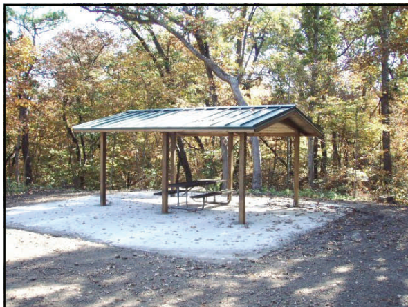
16' x 20' Covered shelter with water and electricity.
