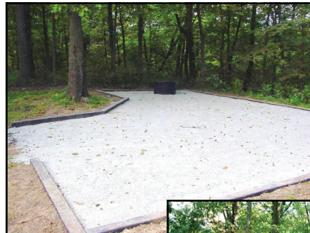
Handicap accessible camping pad.
